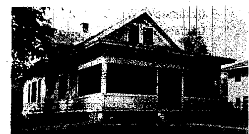
A fine located modern house at 814 Main Street in Wayne, Nebraska. First floor has living room, dining room, kitchen, three bedrooms with closets, and bathroom. Built-in linen closet, desk, bookcases and buffet. Upstairs unfinished, large enough for three or four rooms. Screened-in porch. Full basement. New oil furnace and hot water heater. Garage. Cistern. Nice trees and shrubbery. Location size, 75x150 feet.
